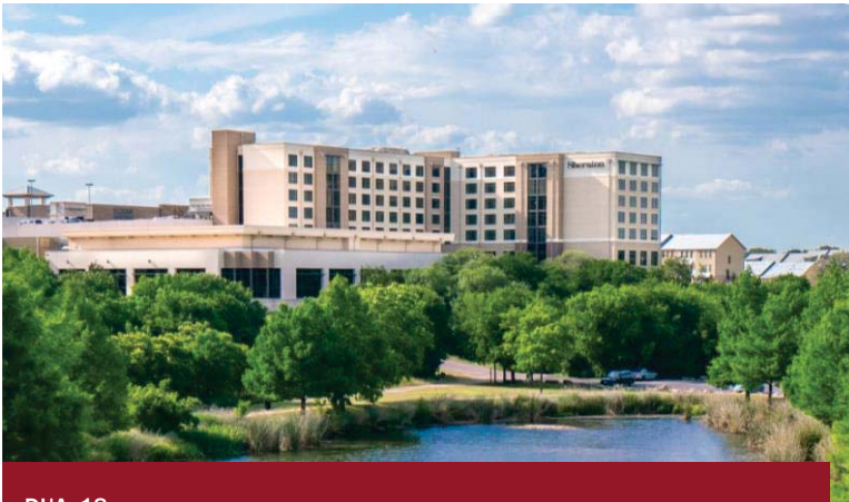
Figure 35. Sheraton Hotel & Conference Center
