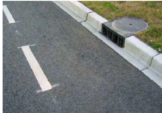
Curb and Gutter
