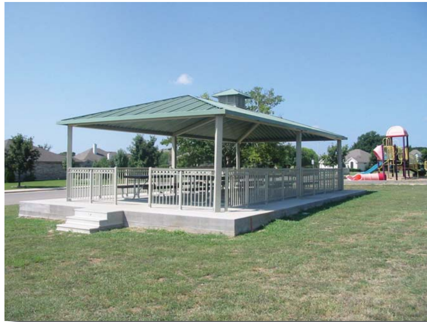
Large pavilion at Katy Crossing Park
